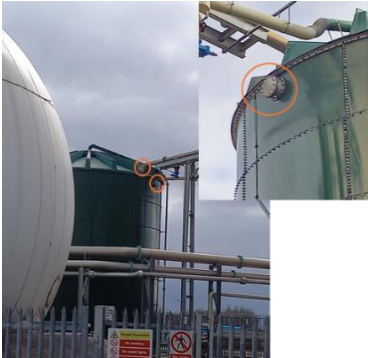
Tank leak
