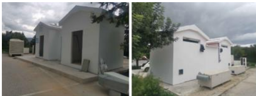
Figure 1: Front and back view of the two demonstration houses in the premises of FORTH
